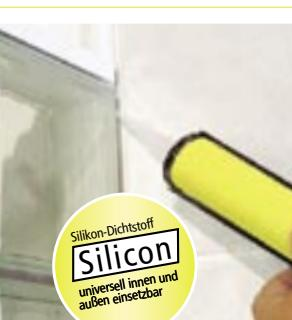
■ Always seal the joints in contact with the wall, floor and ceiling with silicon. Once the finish has been applied clean the surface of the blocks.
